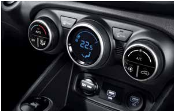
Heating, Ventilation and Air-conditioning Control
