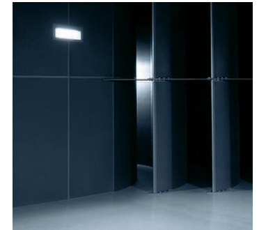
To the rear of the test track, tall hemispherical partitions guide the air flow back in the opposite direction.
